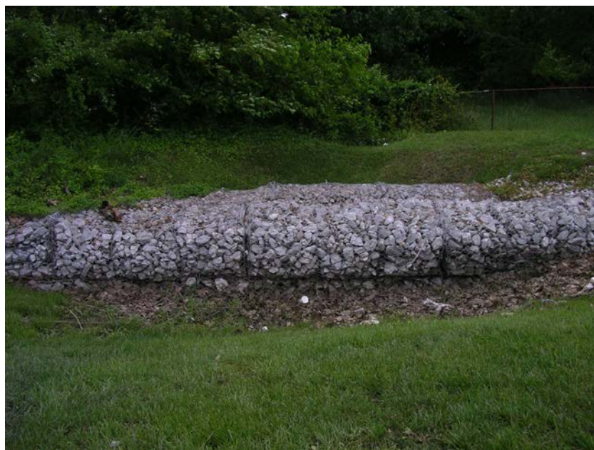
Figure 4-66: A Gabion-lined, Grassy Swale Runs Parallel to the Parking Lot at ISI-A-1633.
