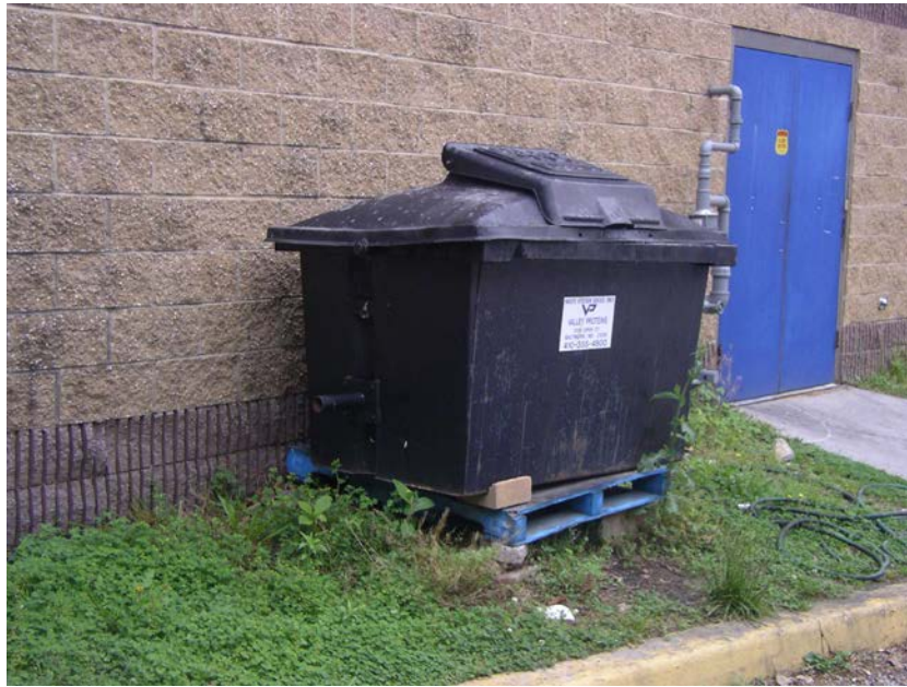
Figure 4-62: A Grease Receptacle Sits Above Porous Pavement at ISI-A-1338. Precautions Should be Taken for This Receptacle in Case of a Spill, Leak, or Puncture, as the Porous Pavement it Sits on Would Absorb any Spills and Allow Them to Seep into the Ground, Eventually Entering Nearby Streams.
