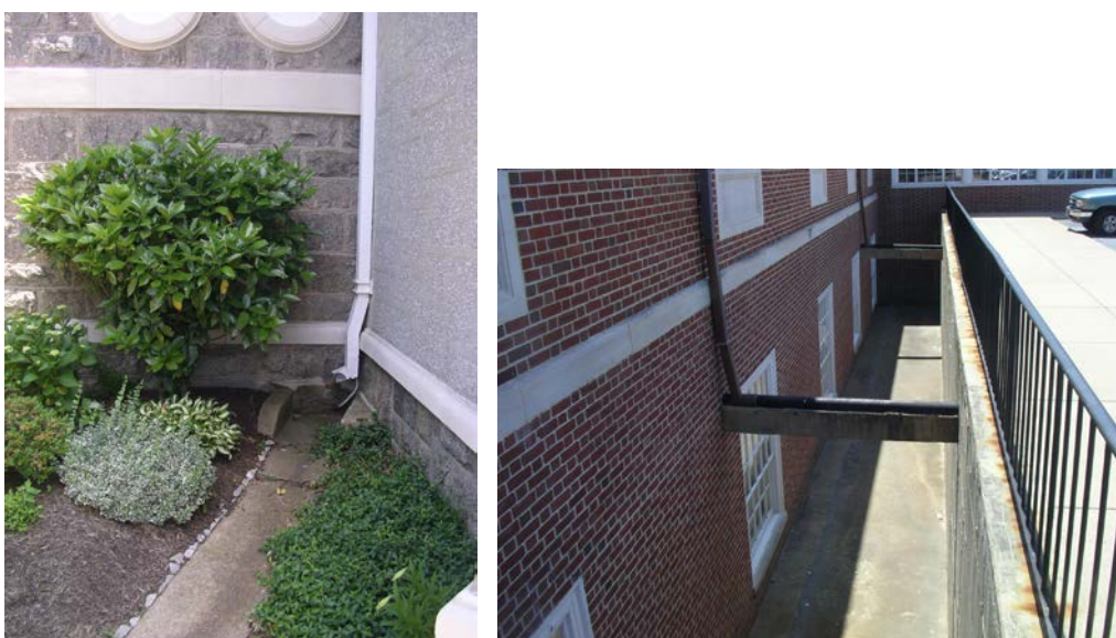
Figure 4-32: Downspouts at ISI-A-916 Could be Redirected to Improve Stormwater Infiltration.
