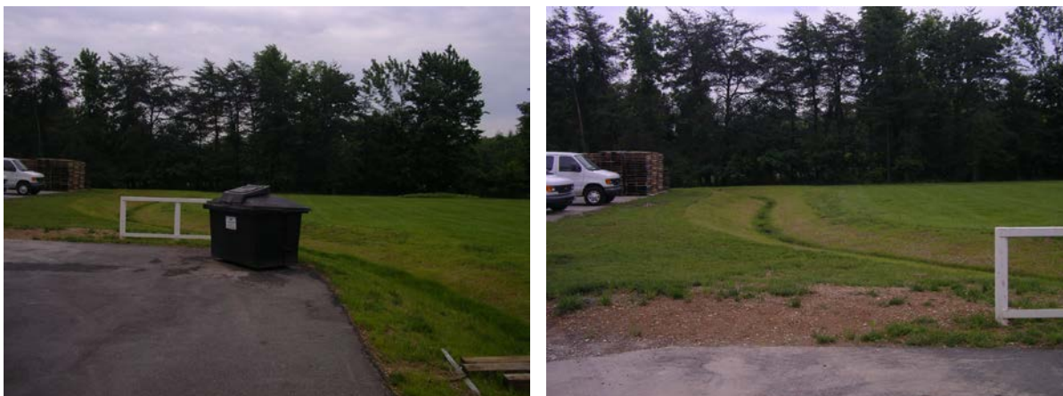
Figure 4-48: A Grease Receptacle Sits Adjacent to a Stormwater Swale, With No Secondary Containment, at ISI-A-1338. Precautions Should be Taken for This Receptacle in Case of a Spill, Leak, or Puncture to Avoid Polluting the Swale and Stream Below.
