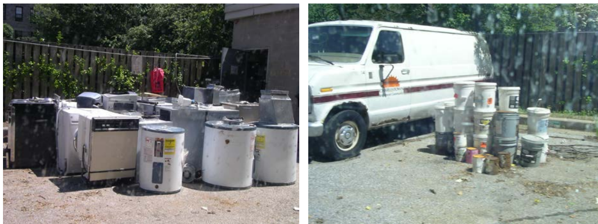
Figure 4-54: Poor Materials Storage Practices Were Observed at ISI-A-1422.
