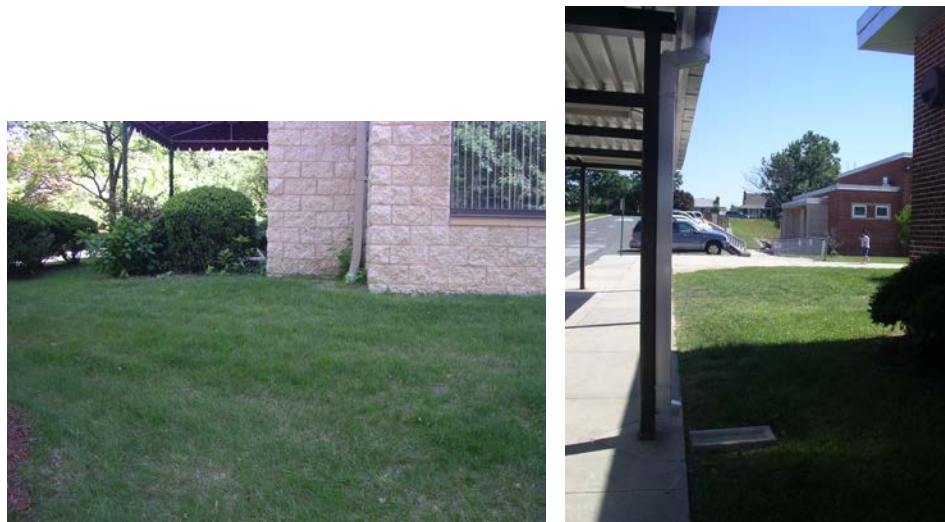
Figure 4-53: Opportunities Exist for Downspout Disconnection and Creation of Rain Gardens at ISI-A-1422 (left) and ISI-A-1439 (right).
