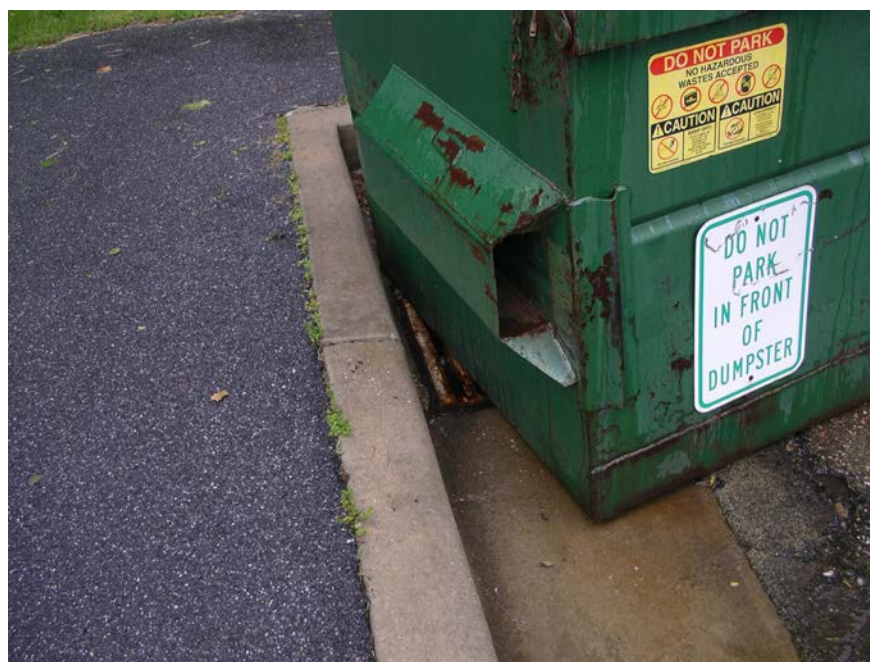
Figure 4-12: A Dumpster Sits Perilously Above a Stormwater Inlet at ISI-A-407.
