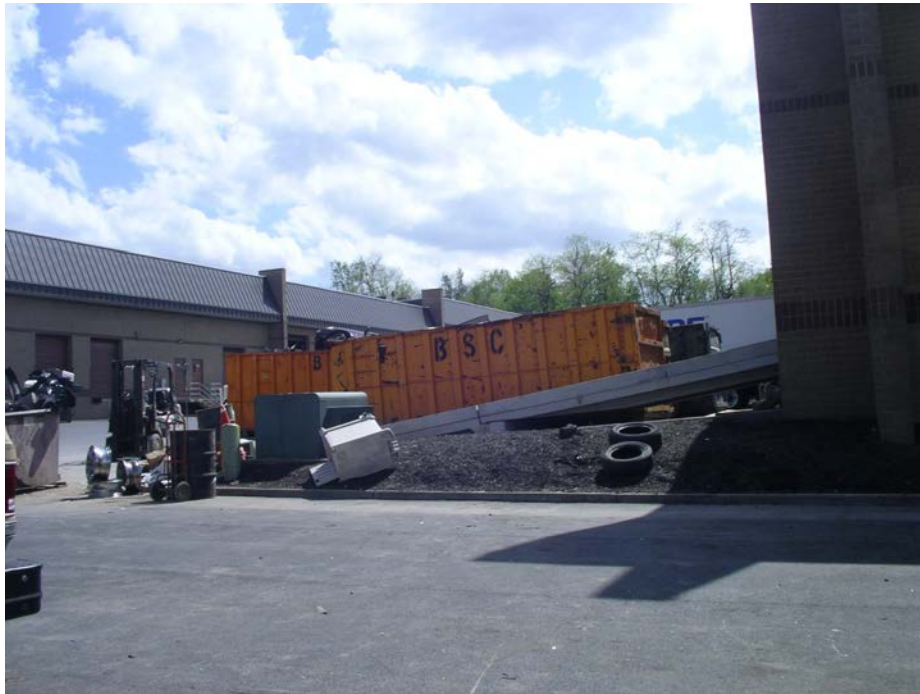
Figure 4-51: Metal Recycling Facility at HSI-A-1416
