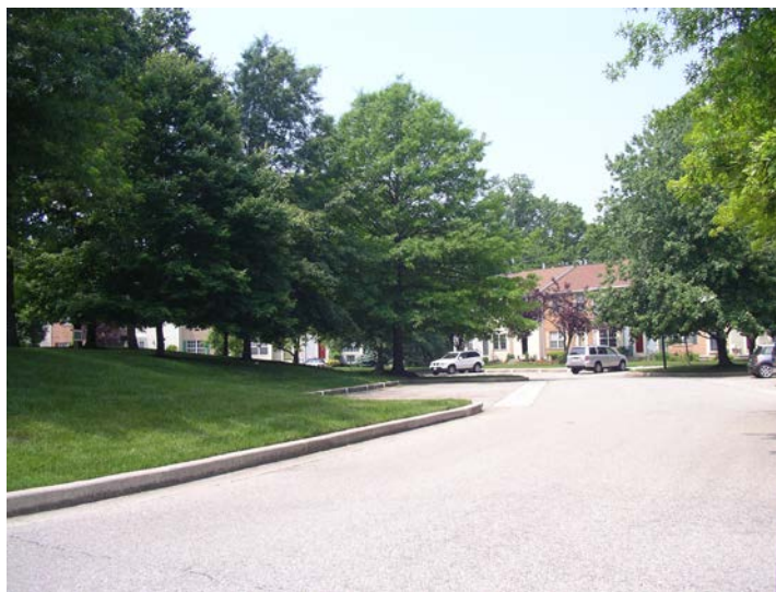
Figure 4-11: There was an Opportunity for Parking Lot Retrofits in NSA-A-1028.
