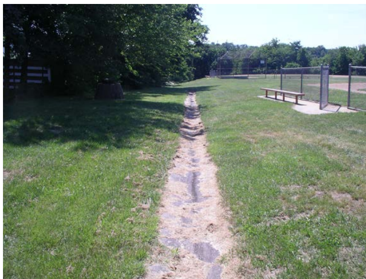
Figure 4-55: Grass Clippings Accumulate in a Concrete Gutter at ISI-A-1439. During Storms, These Clippings Will be Washed Away and Contribute to Nitrification in Downstream Waters. Removal of This Impervious Gutter is Recommended, as it Could be Converted to a Pervious Swale.
