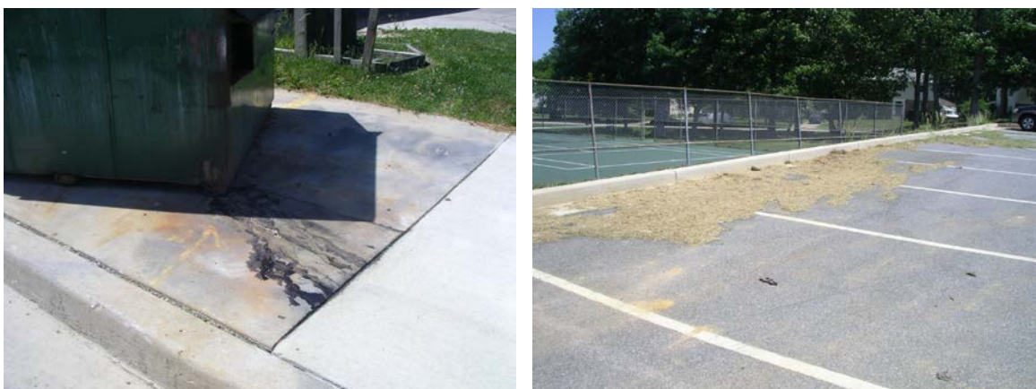
Figure 4-8: A Leaky Dumpster and Excessive Grass Clippings Accumulated on the Parking Lot were Observed at ISI-A-306.
