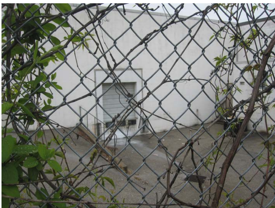
Figure 4-58: White Staining From Loading Dock and 55-Gallon Drums, Both Proximate to Storm Drain at HSI-A-1520
